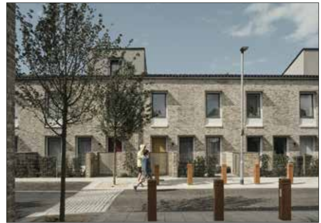
The use of clay bricks and roof tiles provided the perfect low maintenance cladding solutions.
