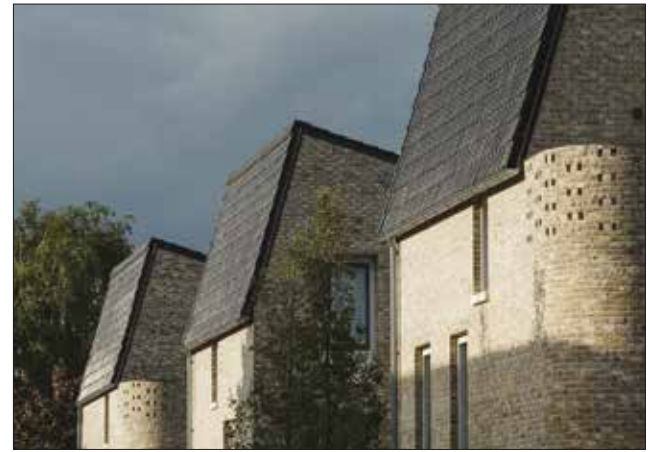
The use of glazed black pantiles and the warm earth colours of the bricks evoked the colours and textures found in the area.
