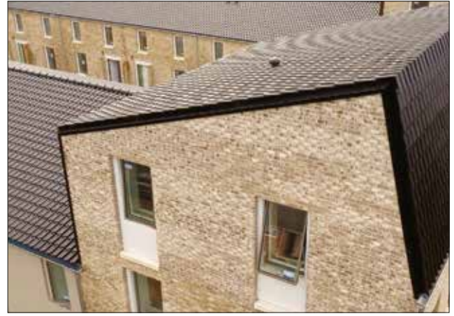
The unique roofing system flows without interruption continuously from eave to ridge.
