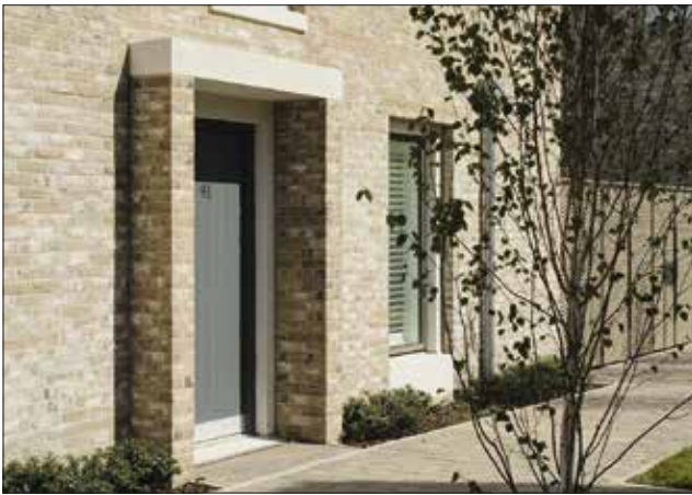
Crest's Belgravia Buff Multi and Grosvenor Multi, a mix of the two brick types created a bespoke and unique blend, now called the Crest Goldsmith Blend which complemented the Victorian terraced housing design.
